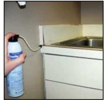
Treat in damp voids harboring German cockroaches.
