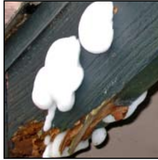
Direct wood injection for pests such as drywood termites, subterranean termites or wood destroying beetles.
