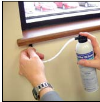
Treat voids harboring overwintering pests such as lady beetles, cluster flies, boxelder bugs, etc.
